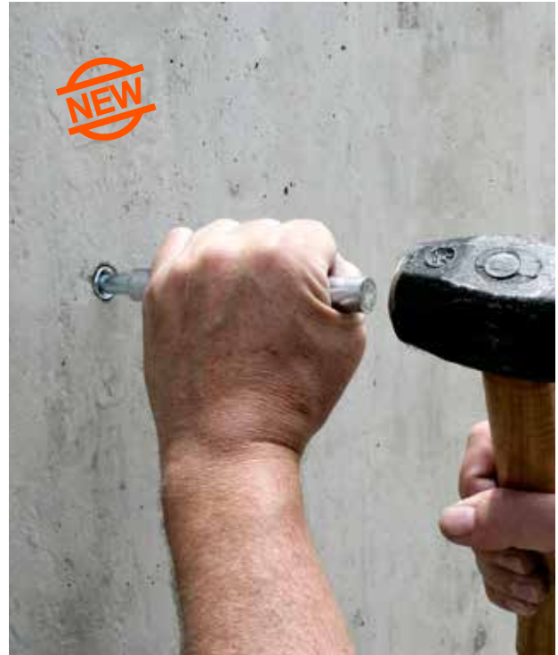
Anchor being set with hand setting tool.
